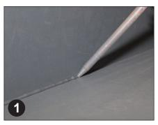
Apply a continuous ‰" bead of Protect-All Rapid Weld at the 90° transition where the Protect-All base sits on the floor.
