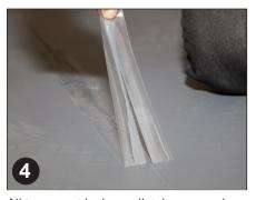
All tape must be immediately removed prior to the Protect-All Rapid Weld curing.
