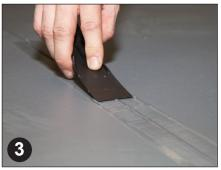
Using the Rapid Floor Seam Finishing Tool, immediately smoth the uncured weld at 20° angle with the bevel facing down. Focus pressure 1" from the end of the finishing tool to leave a thin transparent film on the tape.
