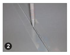
Apply Protect-All Rapid Weld with the dispensing gun at a 90° angle into the prepared groove so it is filled from bottom to top.
