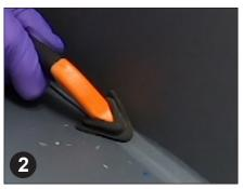
Using the Rapid Radius Finishing Tool, immediately begin to pull across the uncured weld at a parallel angle to create a minimum %" radius transition onto the floor and base.
